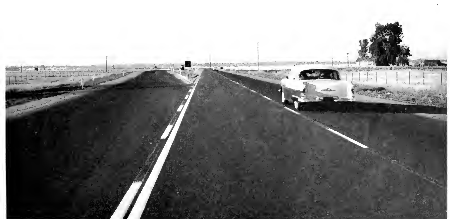
View of section of relocated portion of US 99E between Oroville Wye and Chico
